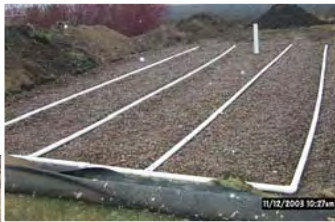
Replacing a septic tank and drain field
