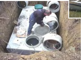
Replacing a septic tank and drain field
